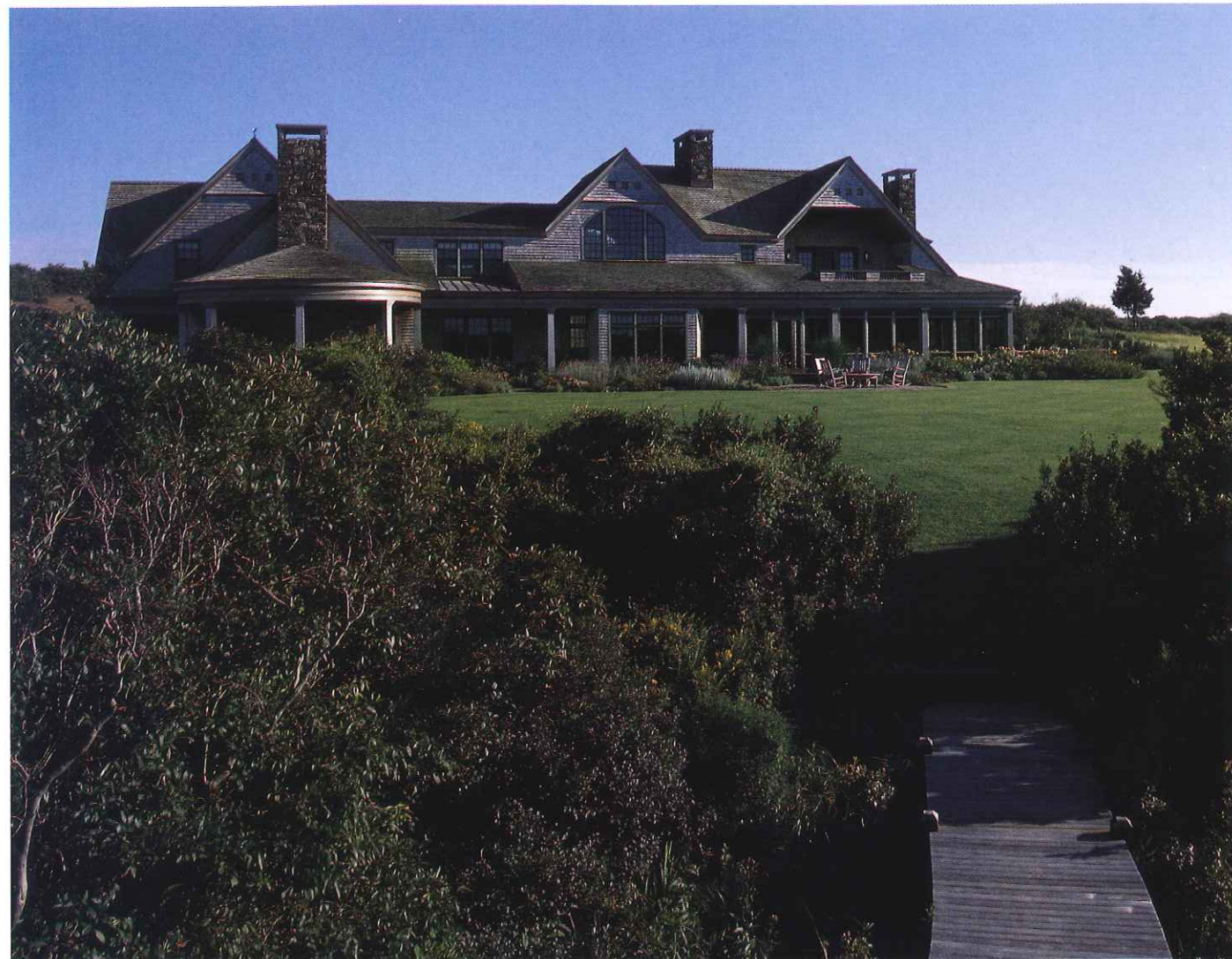
■ Though sheltering 28 rooms, the Meadow house does not dominate the landscape. "In a shingle-style home," says architect Bill McGuire, "a lot of the house is inside the roof. It helps bring down the scale and makes the house feel more intimate."
